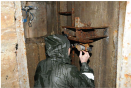
Fig. 3. A measuring position of pendulum wire displacements using a mechanical device
